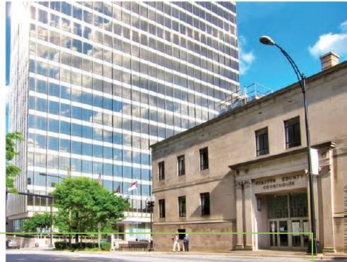
Old County Courthouse & Winston Tower
